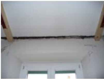
LACK OF CONNECTIONS
