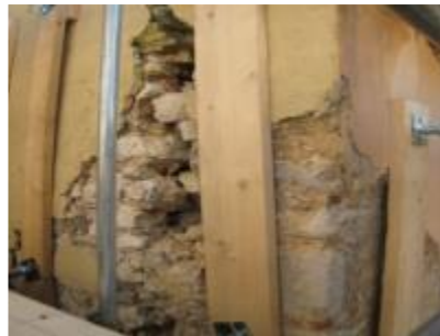
INSUFFICIENT MASONRY QUALITY
