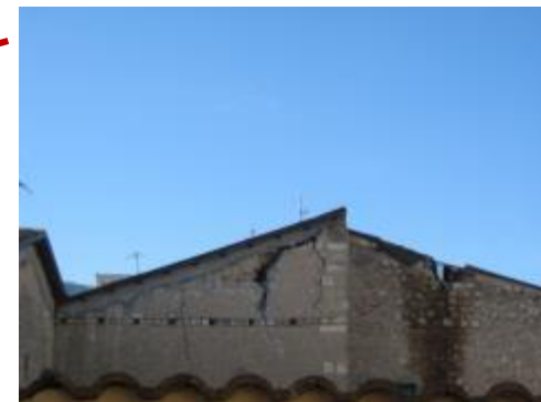
WEAKENING OF MASONRY
