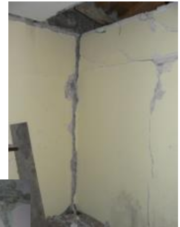
LACK OF CONNECTION BETWEEN ORTHOGONAL FLOORS
