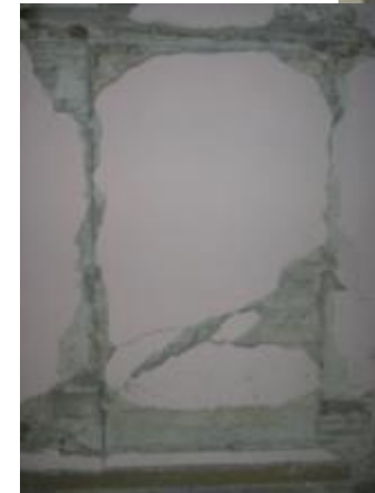
LACK OF CONNECTION BETWEEN ORTHOGONAL FLOORS
