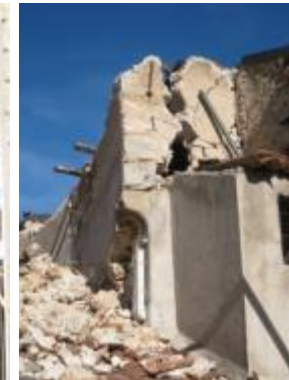
OVERTURNING WITH INVOLVEMENT OF THE WEDGE
