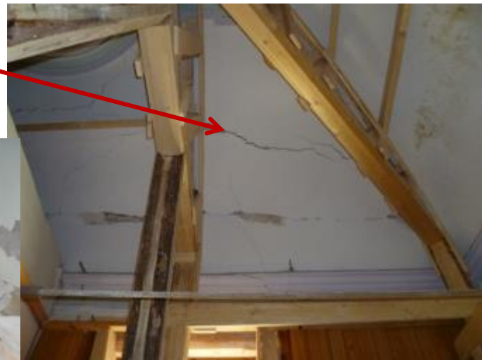
CRACK AT THE SPRINGINGS
